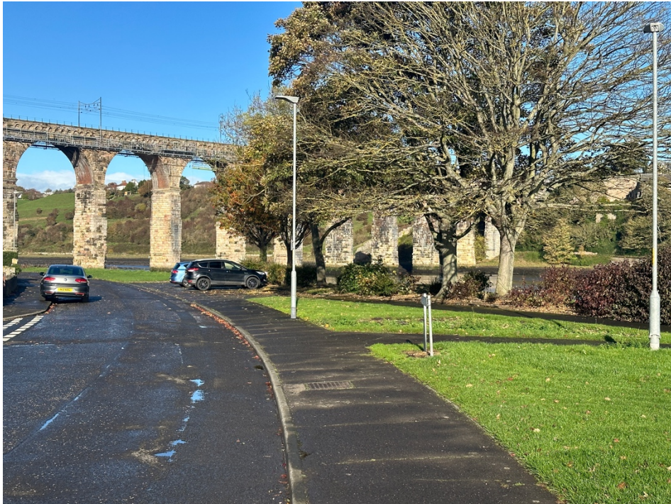
Riverside in Tweedmouth: A more coordinated approach would be helpful, based on a design code.
