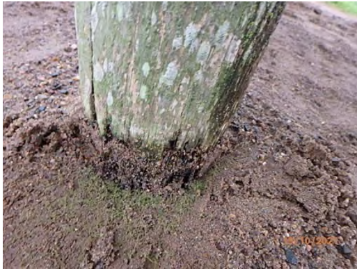
Timber posts are rotting in the ground
