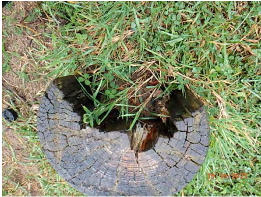
Short Post Steppers are rotting
