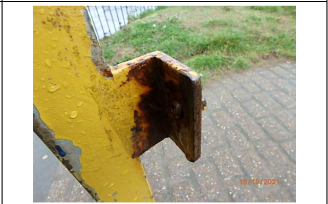
Crush point between fence and gate
