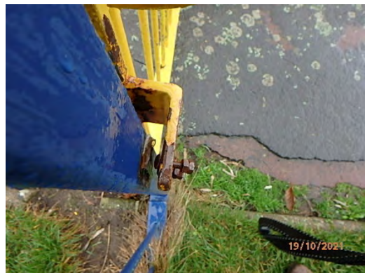
Crush / slam hazards
