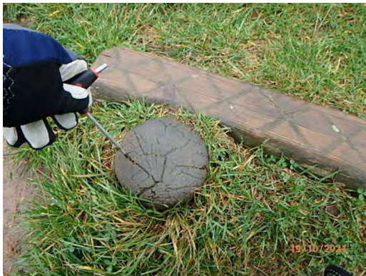
Short Post Steppers are rotting
