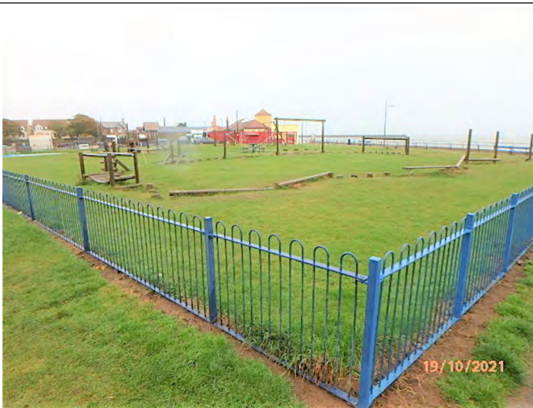
SITE: SPITTAL PAVILION PLAY AREA, SOUTH GREENWICH ROAD, SPITTAL, BERWICK UPON TWEED. TD15 1RW.
