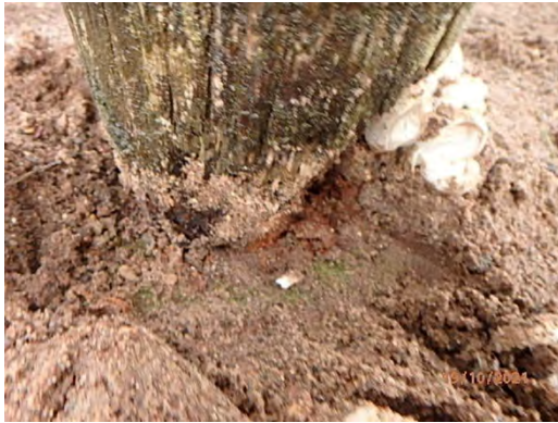
Timber posts are rotting in the ground
