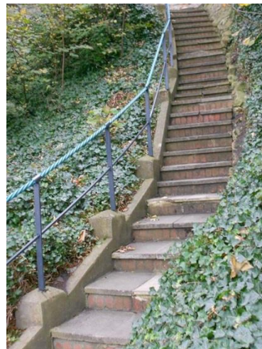
Photo 4 Style of replacement handrail
